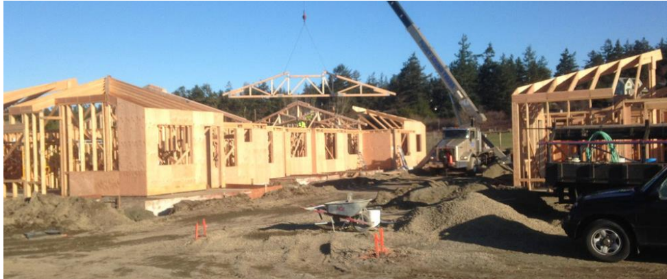
Figura 23 - Construção da Quimper Village Senior Cohousing
